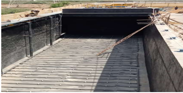
Design, Engineering and execution of complete mix activated sludge process for Artistic Milliners Textile AMPQ effluent treatment plant ETP 55 m3/hr
