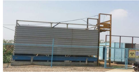
Trickling bio filter STP, 100,000 GPD Karachi , Pakistan
