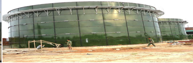
Design, Engineering and execution of complete mix activated sludge process for Artistic Milliners Textile AMPQ effluent treatment plant ETP 55 m3/hr
