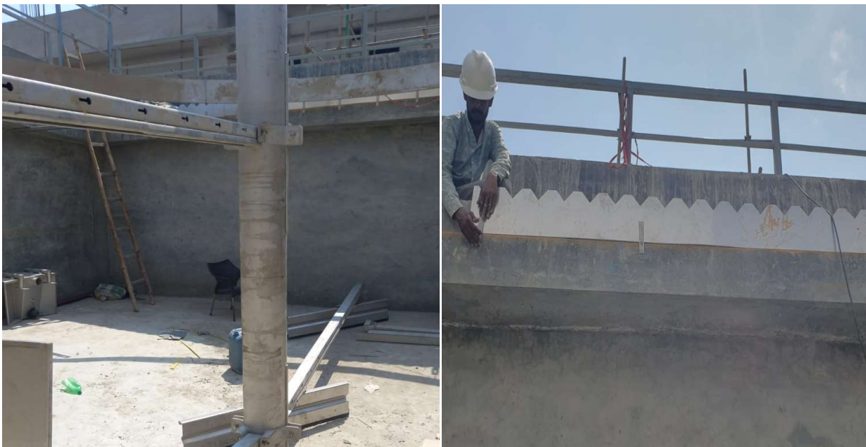
Design , fabrication and installation of fix bridge clarifier 8 meter dia
