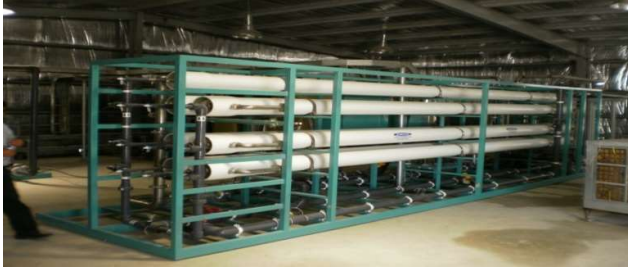
Naduro Sugar Power plant 47 m3/hr RO + CEDI 2011
